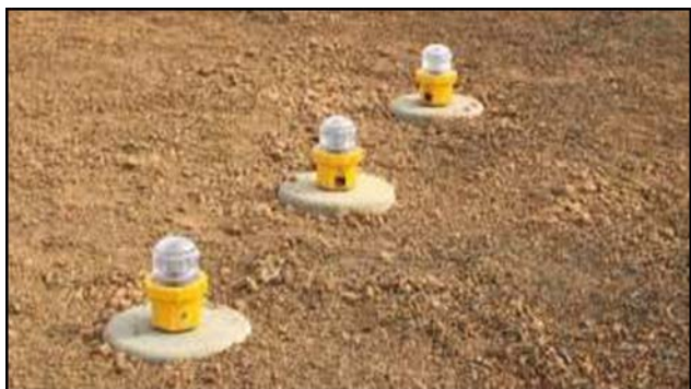
(New LED Lights Installed at the Air Strip – July 2018)
