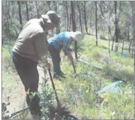
Below – Wayne Zadow and Kath Mathwin digging holes for the sign posts.
