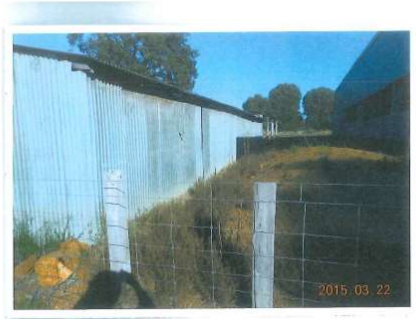
WALL WILL GO FULL LENGTH OF THIS WALL.
