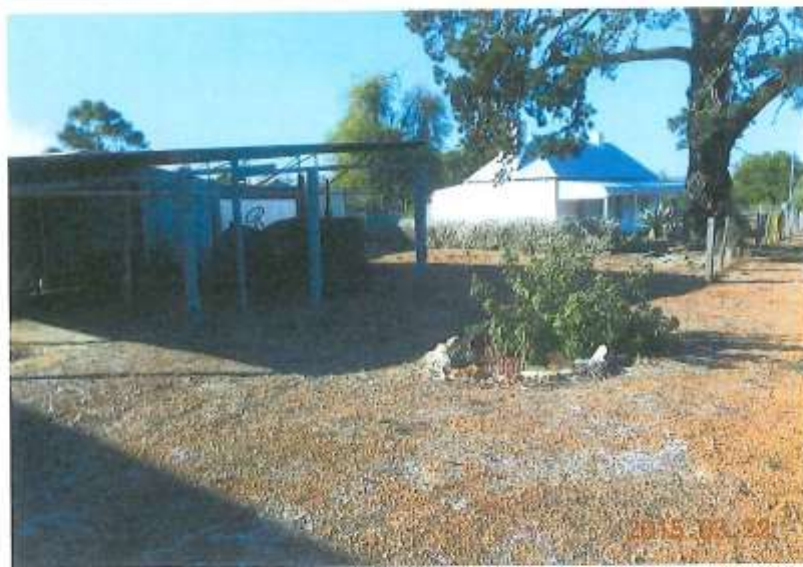
ELVERD COTTAGE, OLD MACHINERY SHED SHOWING DISTANCE FROM COTTAGE.
