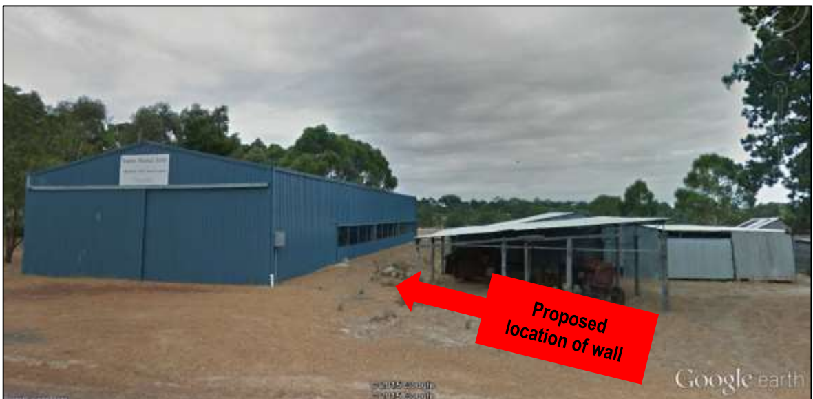
Proposed retaining wall site Lot P2 Soldier Road, Kojonup (Image taken from Soldier Road on Google Earth)
