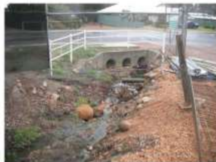
Downstream drain crossing under Elverd Street.
