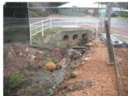
Downstream drain crossing under Elverd Street.
