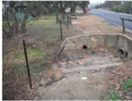
The inlet to the drain road crossing under Honner Street.
