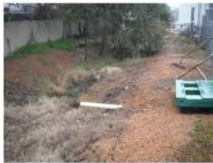
View of open drain adjacent to Co-op yard.
