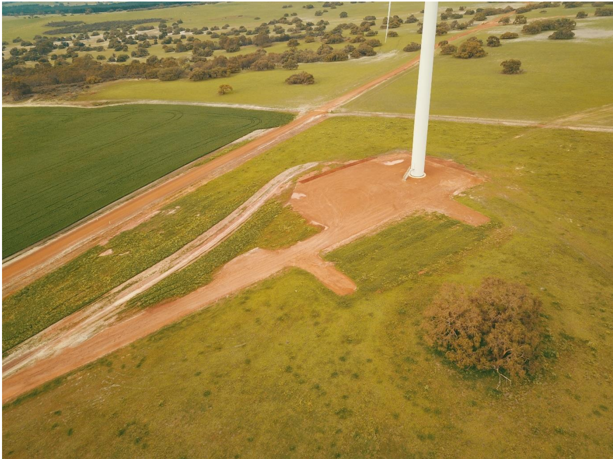
Plate 1: Typical turbine, a clear base within open land (pasture), retained crane pad and access track.
