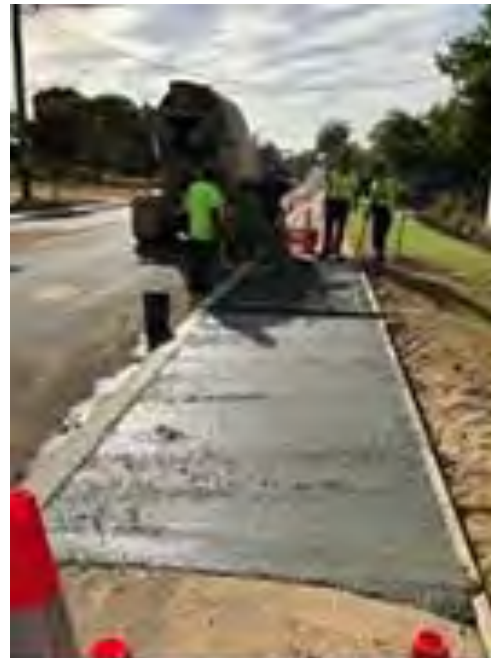
Kerb laying - Spring Street
