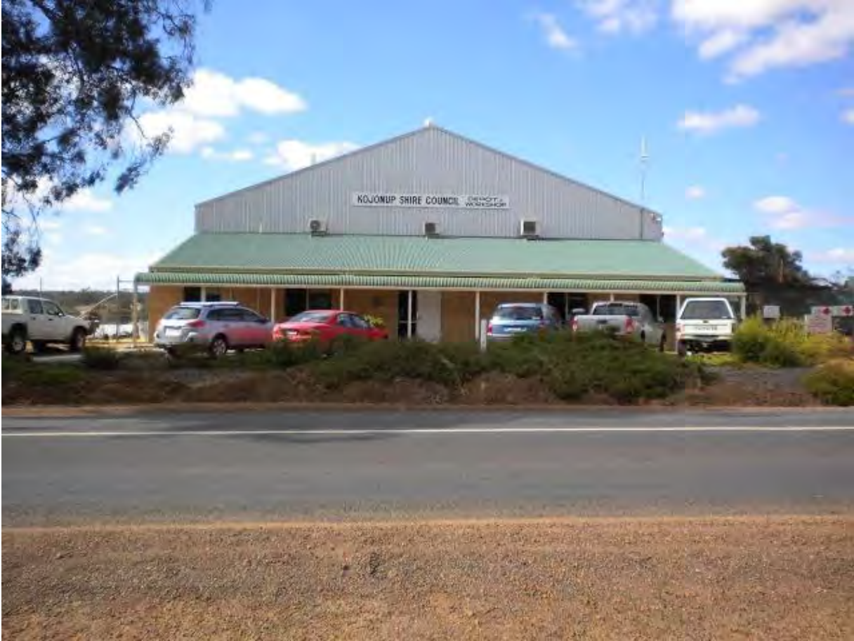
Shire of Kojonup Depot
