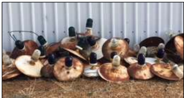
(Pile of Old Lights that were taken out)
