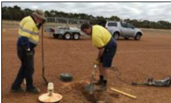
(Old Lights being taken out at the Air Strip)
