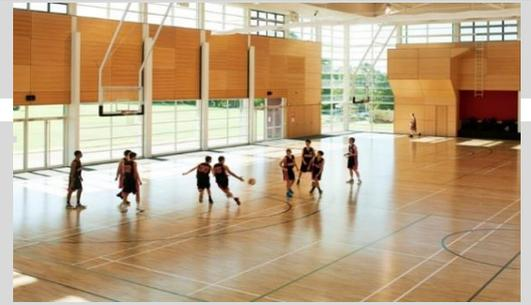
Helsinki is a state of the art system which offers considerable cost savings from a life cycle perspective. This type of timber flooring will not require recoating for approximately 10 to 15 years, after this it must be annually recoated just as any other timber system. Other advantages are higher shock absorption, moisture stability, increased durability of top layer and factory engineered finish. This system is FIBA 1 Certified
